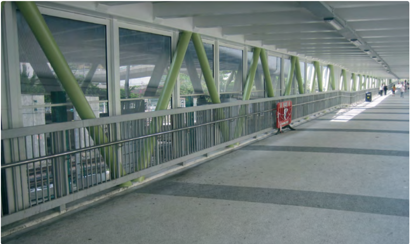
Project: Kowloon Bay MTR (Metro Station) - Hong Kong, China (2008) | Barrier Glazing: PALGLAS® 20mm Grey
