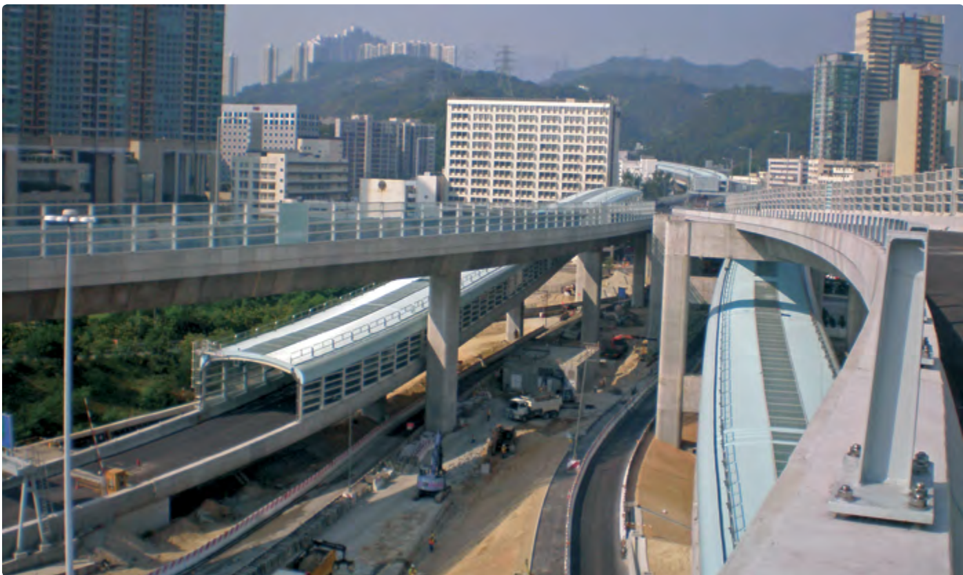
Project: Lai Chi Kok Viaduct - Hong Kong, China (2006) | Barrier Glazing: PALGLAS® 15mm & 18mm Clear & Light Blue
