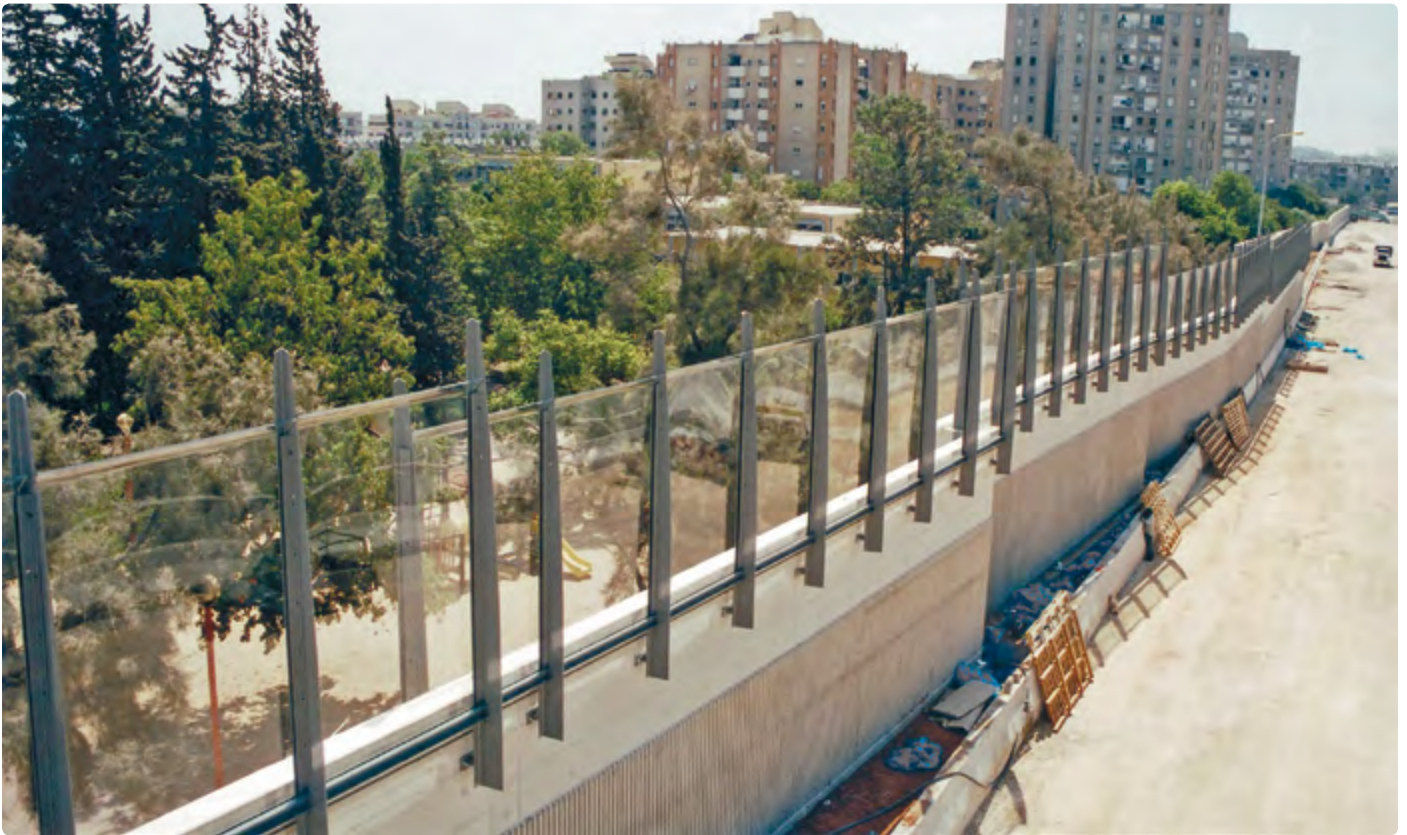
Project: Ayalon/Holon Interchange - Israel (2003) | Barrier Glazing: PALGLAS® 20mm Clear
